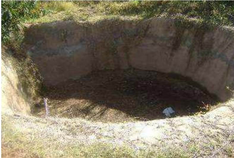
Fig 4.6.ponds lined by combining cement, sand and 'kuyissa'(photo by author)
