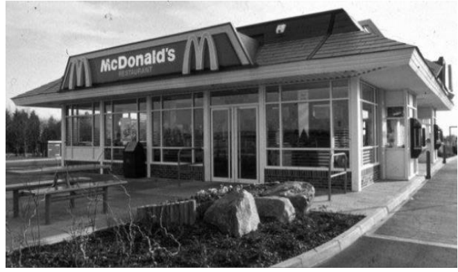
Figure 2.3: Fast-food restaurant in UK, which is fitted out before delivery to site (RM Lawson, 1999)
