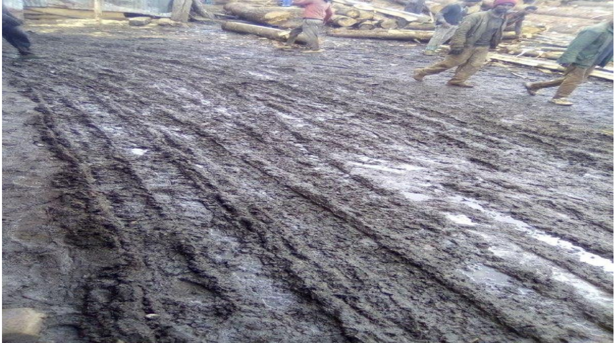
Figure 6: Road in Tsion industrial park wereda 9, 2022
