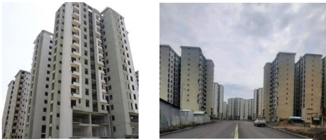
Figure 4.6 Bole Bulbula 40/60 condominium housing project
