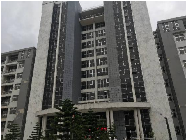
Figure 4.2 Image of Bole sub city building project
