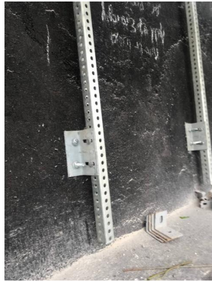
Figure Error! No text of specified style in document..7 Installation of stone cladding at children and youth theatre
