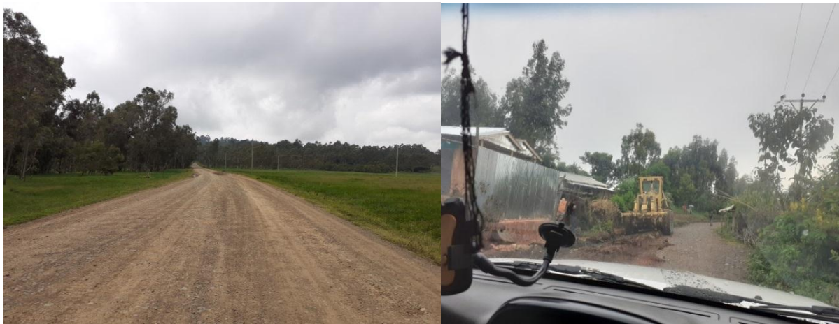
Road construction in Chanchu Woreti
