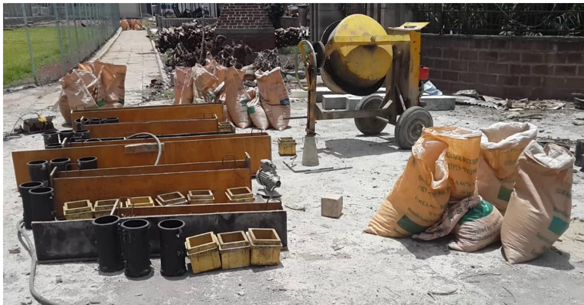
Figure 3-3: Batching and preparation of concrete ingredients before mixing
