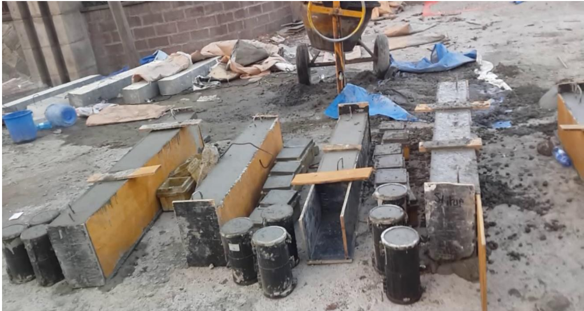
Figure 3-9: concrete casting on beam specimens and representative samples
