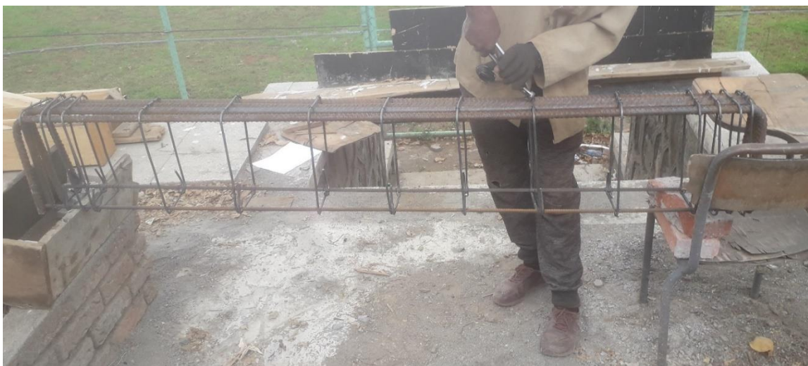
Figure 3-7: Reinforcement cage preparation
