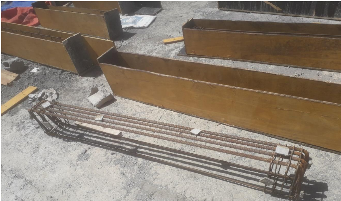
Figure 3-8: Formwork preparation and concrete cover assembling
