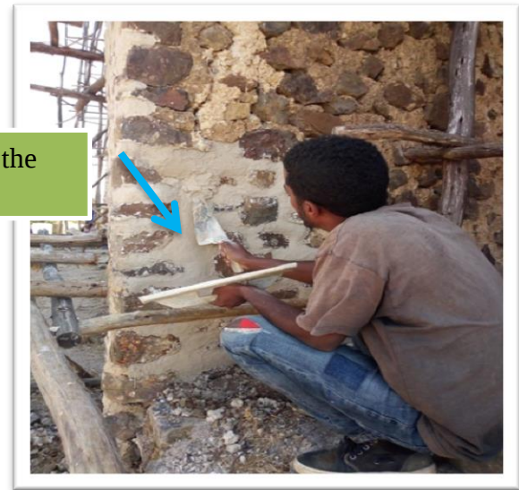
Figure 3.21 Mortar used in repairing the Castle (Photo by Kedir 2018)
