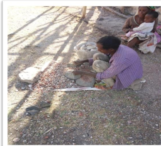
Figure 3.20. A man pounding coarse limestone debris (left figure), and a man mixes limestone powder with coarse limestone debris to make it ready for conservation (right figure) (Photo by Kedir 2018)
