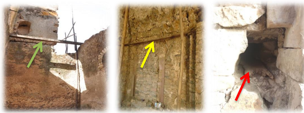
Figure 4.3. Materials used to construct a) Wood beams at Guzara Castle (the left figure), b) Metals at Bahri Gemb (the middle figure), and c) Wood beams at Debsan Ginb (the right figure) (of the Monuments) (Photo by Kedir 2018)
