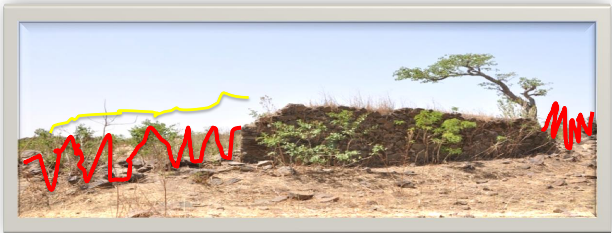
Figure 3.30 Destructed Enclosure of the Church (Photo by Kedir 2018)
