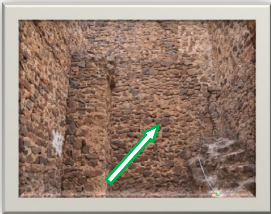
Figure 4.14: Deterioration of the Mortar and decay of the Palace of Guzara (Photo by Kedir 2018)
