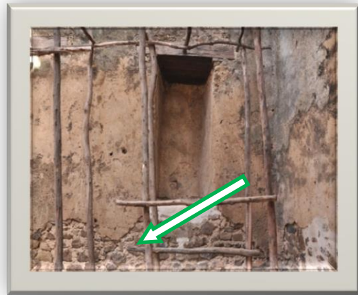
Figure 4.14: Deterioration of the Mortar and decay of the Palace of Guzara (Photo by Kedir 2018)
