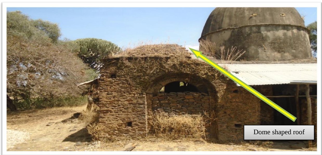
Figure 3.53 A part of the Bahri Ginb roof, providing a hint how the original roof of the building seemed like (Photo by Kedir 2018)
