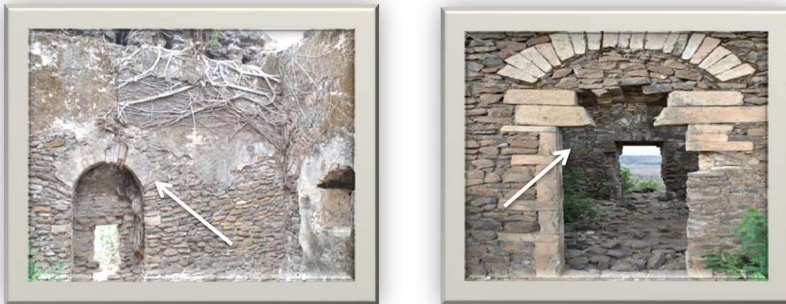
Figure 3.38 Arched Windows (left figure) and Doors (right figure) (Photo by Kedir 2018)
