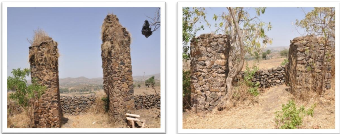
Figure 3.10. Western gates of the Palace (view from inside): better preserved but grasses are grown on it (left figure), and gate on destruction (right figure) (Photo by Kedir 2018)
