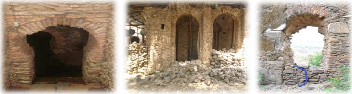
Figure 4.8. Lime mortared Brick of Arches found in Aksum (left figure) (after Werku 2015) and a similar architecture in Bahri Gemb (middle figure), and in Debsan Gemb (right figure) (Photo by Kedir 2018)
