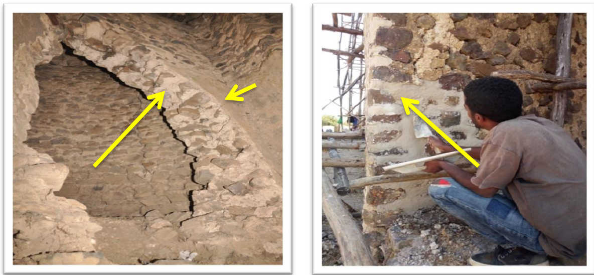
Figure 3.22 Conservation difference: old building, very compacted, well done where much amount of lime mortar used, (left figure), and wall conserved slightly by lime mortar (right figure) (Photo by Kedir 2018)
