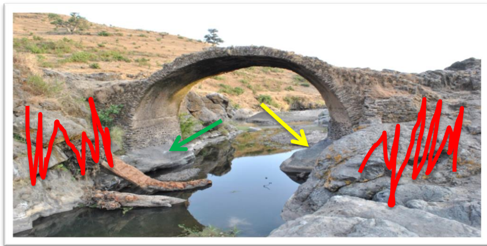
Figure 4.2. Shows the basement Granite rock over which Gobatit Dildiy was built (Photo by Kedir 2018)
