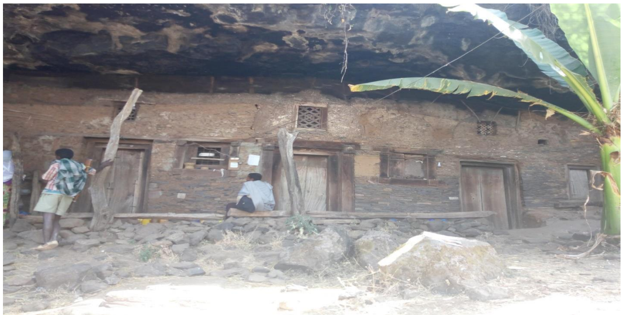
Figure 3.62. Washa Endrias Cave Church, its front view (Photo by Kedir 2018)
