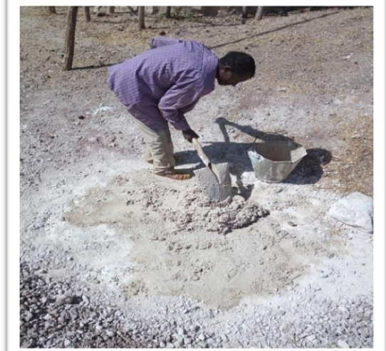
Figure 3.20. A man pounding coarse limestone debris (left figure), and a man mixes limestone powder with coarse limestone debris to make it ready for conservation (right figure) (Photo by Kedir 2018)
