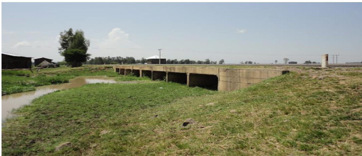
Plate 3-3: Marza River road crossing box culvert (BRL Ingenerie, 2015)
