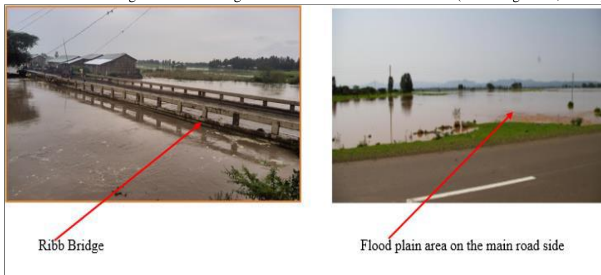
Plate 3-1: Flooding at Ribb Bridge and Road Side Flood Plain (BRL Ingenerie, 2015).
