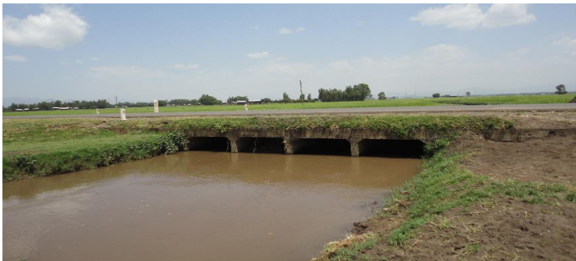
Plate 3-2: Sheni River road crossing box culvert (BRL Ingenerie, 2015).
