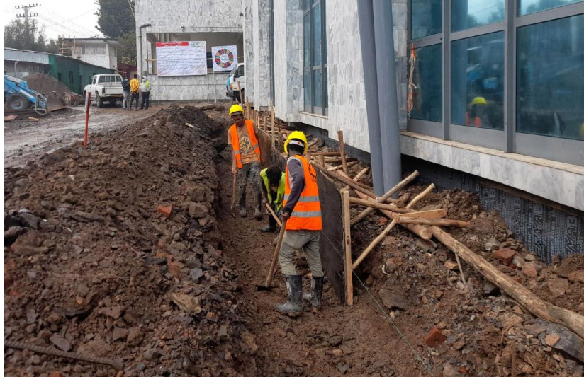
Figure1. 1 ECWC workers at AAPC maintenance project site (Field survey, 2021)
