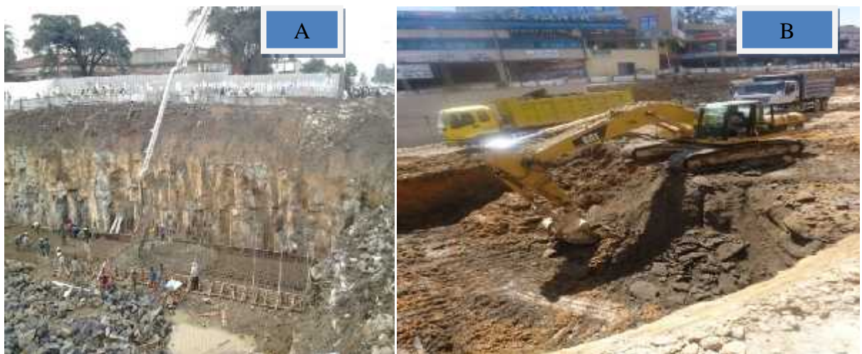
Plate 1.1 Natural subgrade excavated ignimbrite (Plate-A) and highly weathered tuffaceous material (plate-B)
