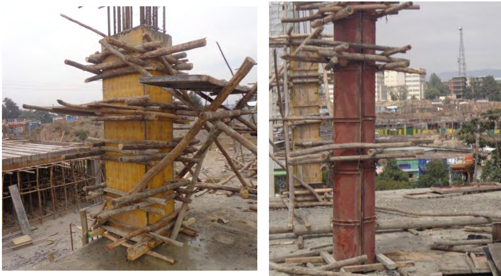
Fig. 2.16 Column formwork construction systems at Sengatera 40/60 projects
