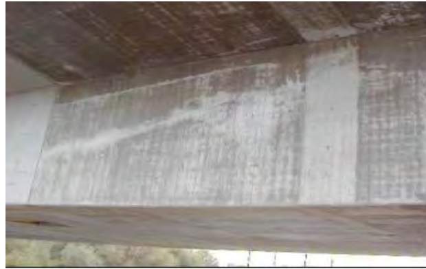
Fig. 2.14 The variation in the grey shade of concrete due to the absorbency of the timber formwork sheathing. (Source: Doka 2008)
