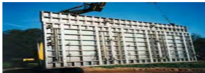
Fig 2.8 Gang formwork system (WTF, Forming systems catalog, 2011)
