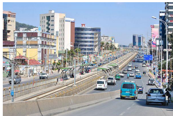
Figure 2.4 At grade LRT
