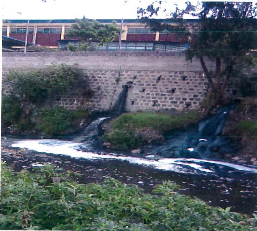
Picture 2 Batu tannery wastewater discharged to little Akaki River mismanaged at source.
