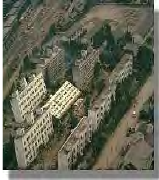
Kawagishi-cho apartments sank in and tipped, Niigata, Japan, 1964
