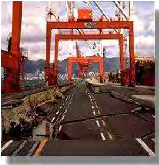
Lateral displacement of quay wall, Kobe, Japan, 1995
