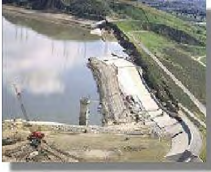
Sanferando dam failure [12]
