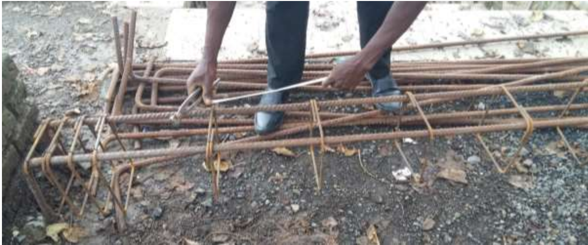
Figure 3.7 : Rebar preparation
