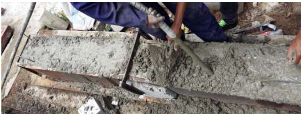
Figure 3.12 : Casting Concrete in Metal formwork
