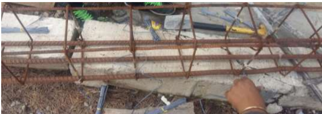
Figure 3.9 : Strain gauge installation for B2C80
