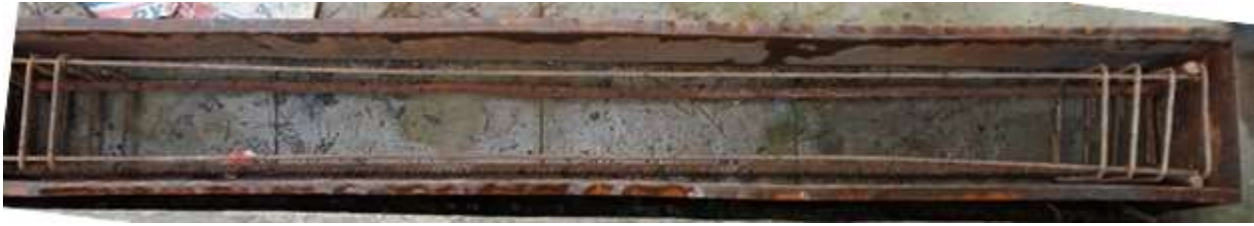
Figure 3.10 : Reinforcement cage placement in formwork
