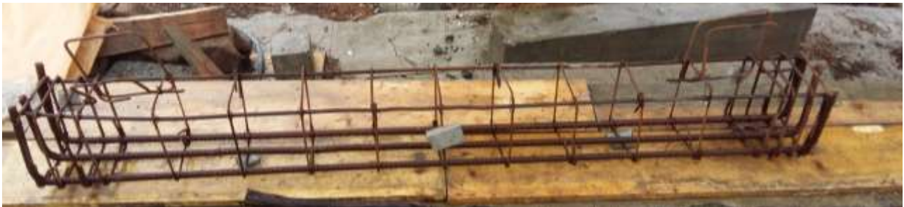
Figure 3.8 : Reinforcement cage for Type 2 Beams
