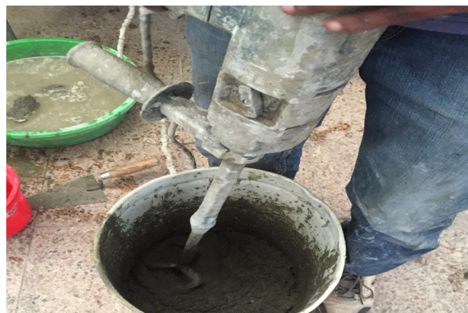
Picture 2: High speed shear mixing of CLC
