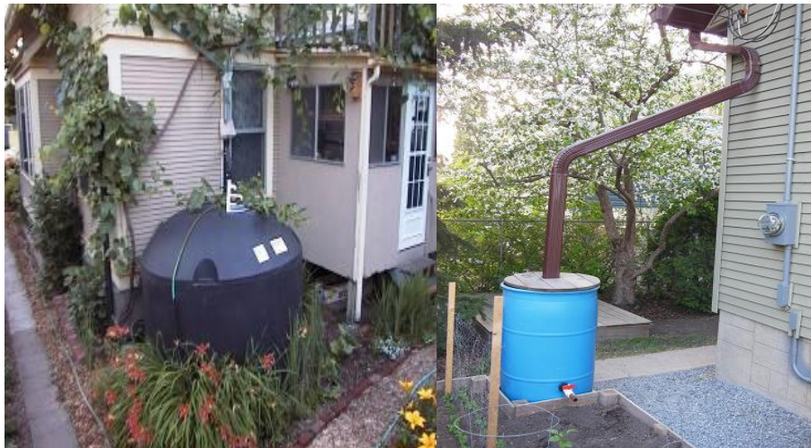
Figure 2: Rainwater harvesting systems
