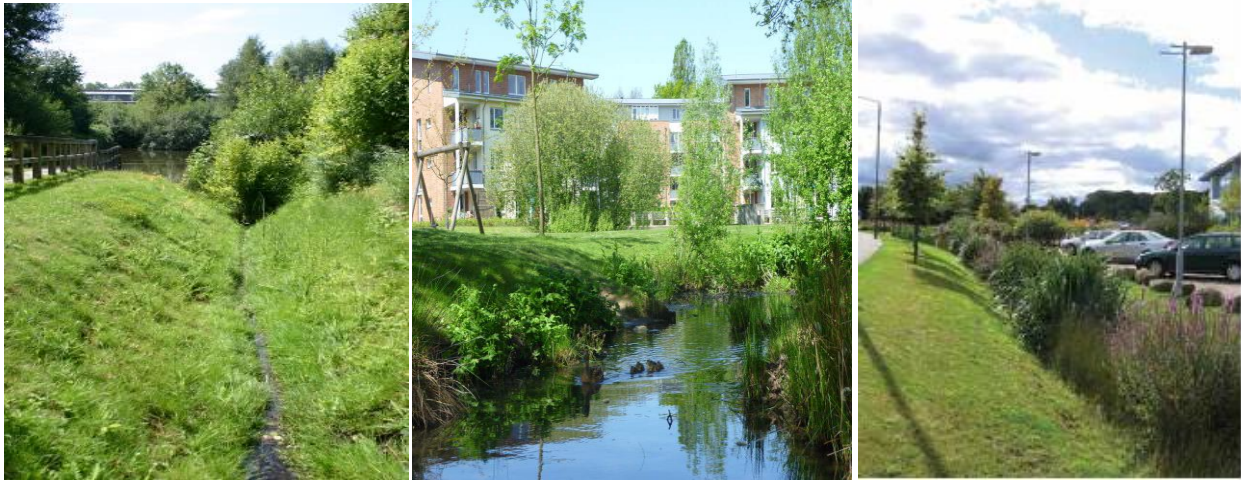
Figure 5: Vegetation Swales along gorges and roads
