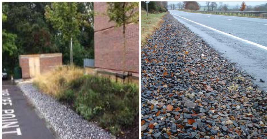
Figure 6: Infiltration trenches along roads, Adopted from ( Woods, 2015 )
