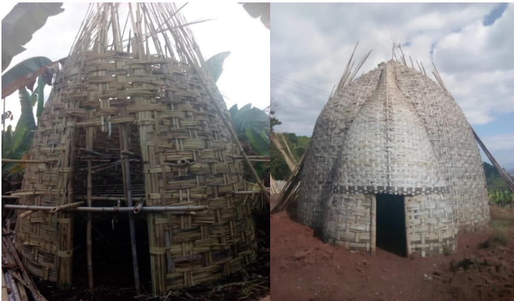
Figure 8 Dorze houses in early stage of building (photo by the researcher, 2018)
