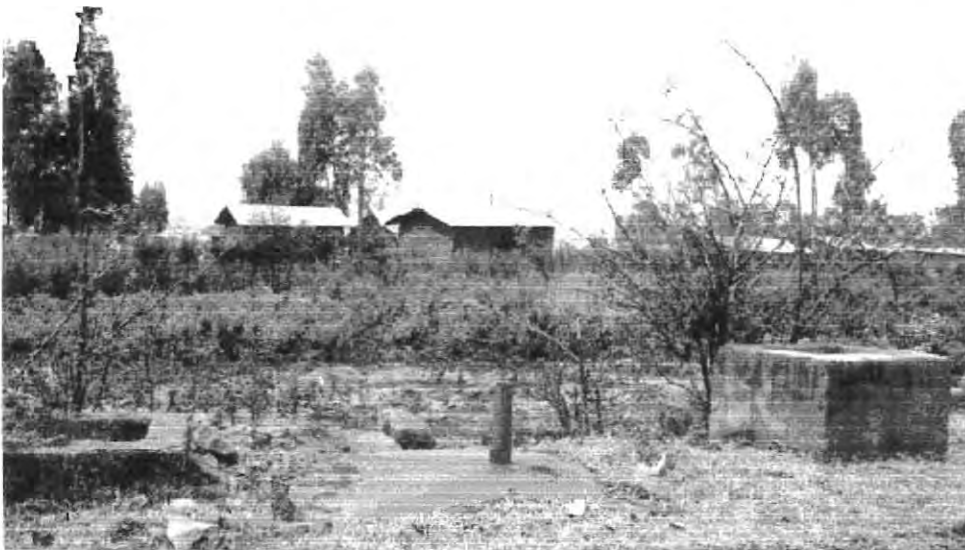
Figure 5.2 Status of Biogas Digester Found at Subshengo Village
