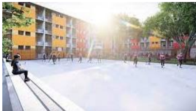
Fig 18: Hawassa Village Workers Dormitory project
