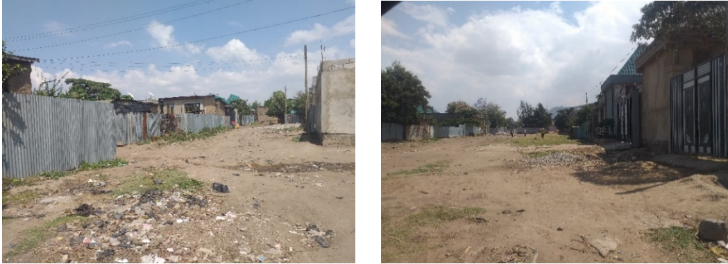
Fig 34: Condition of access roads at 'Tilte' Kebele
