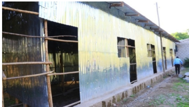
Fig 16: housing for poor
