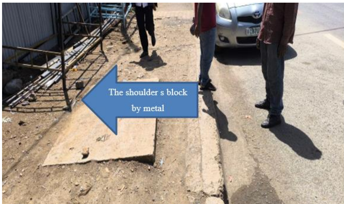
Figure 13 Shoulder cleanness and barrier for road users
