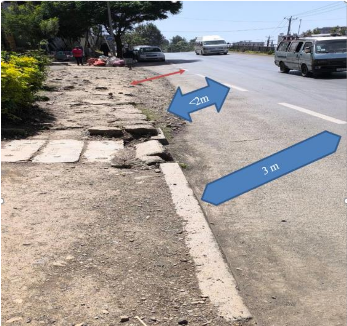
Figure 6 Discontinuities in “through” lanes and unsafe “trap” lanes are identified
