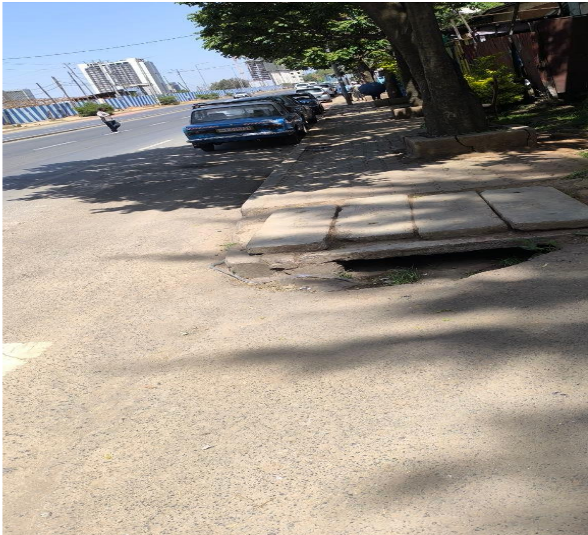
Figure 8 Road side infrastructure
