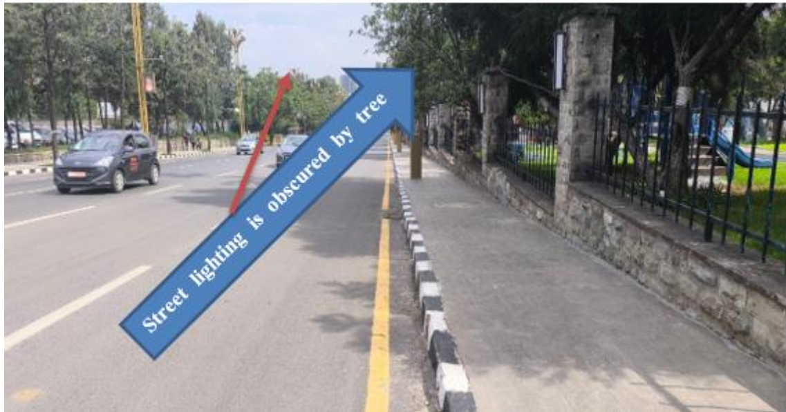
Figure 17 Street lighting is blocked or obscured by tree branches
