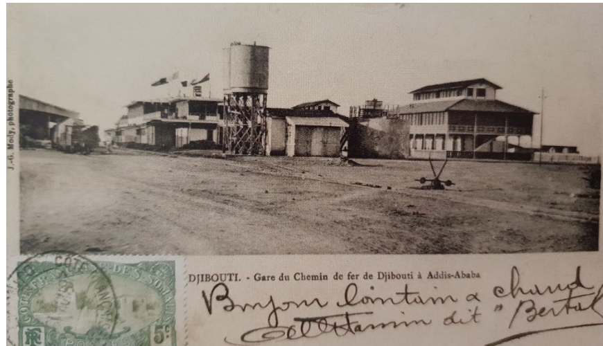
Figure 2-8: Djibouti, the railway station of CIF
