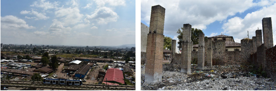
Figure 2-29 Left- Areal view of the settlement of the Federal Police Camp in the Customs Compound, Right- Burnet Warehouse Building [Burned somewhere in between February and June of 2017] Source: Taken by Writer on December 2019
