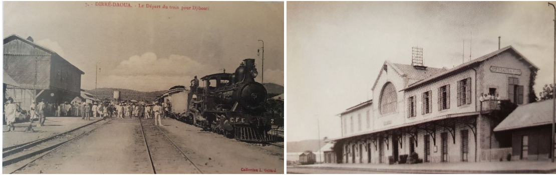
Figure 2-11: The terminal building in Dire Dawa, first wooden [picture on the left] later changed to stone [picture on the right] in the 1910's
