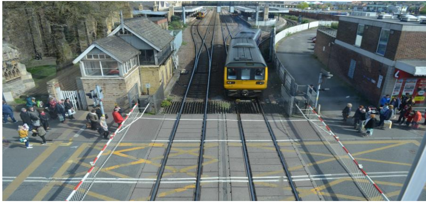
Figure 3-6: User Worked Crossing with Miniature Warning Lights image[52]
