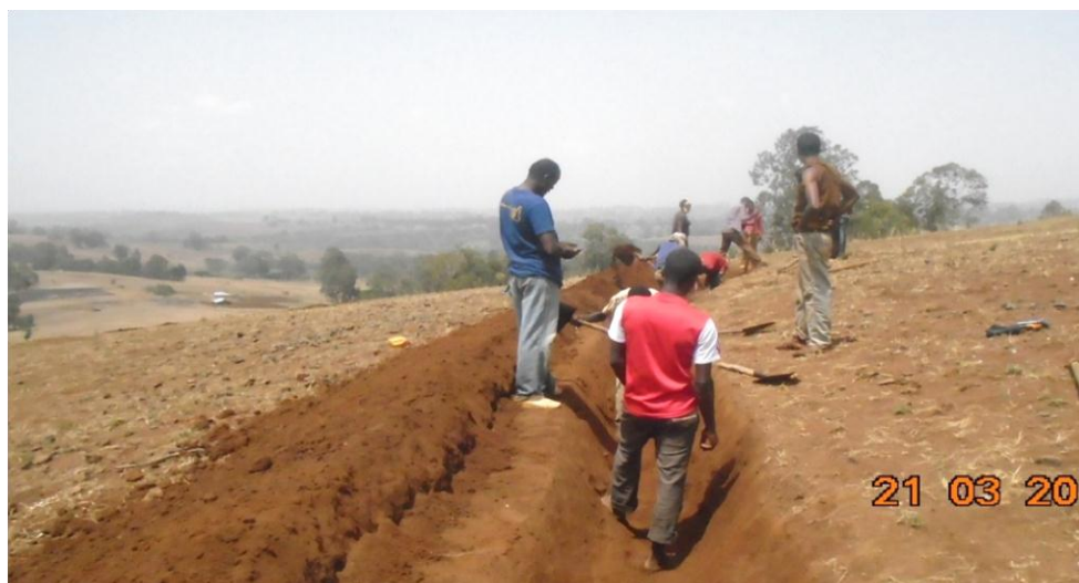
Plate 4. Observation to ongoing work done to maintain damaged land
