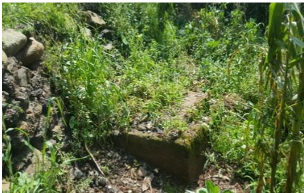
Asko Anaerobic baffle reactors treatment
