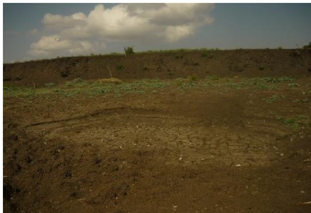
Plate 4.1: Pond constructed with out silt-trap
