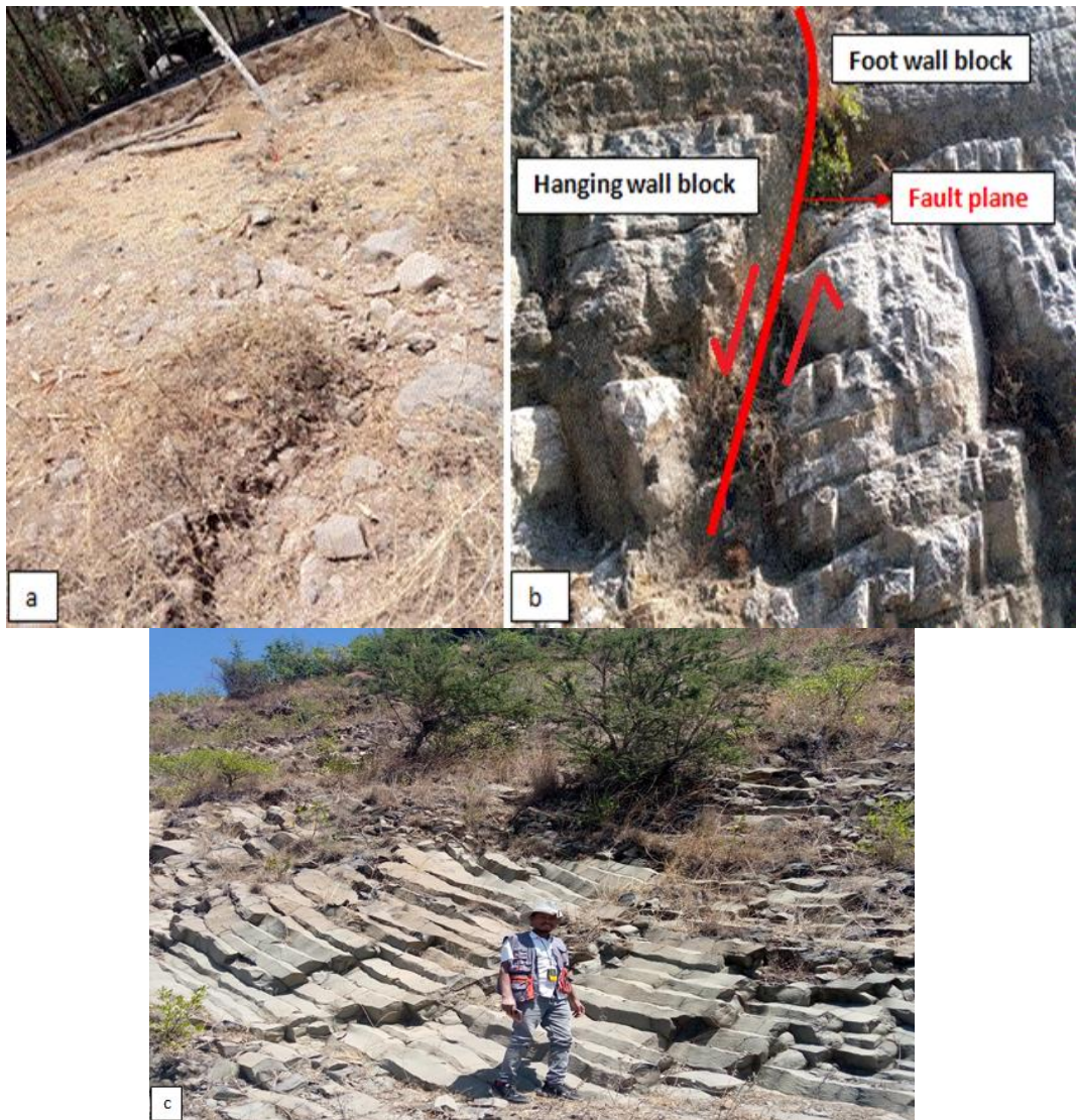
a) Ground crack on the Church compound in Kurar village, b) Normal fault on gypsum bed & c) columnar jointed basalt
