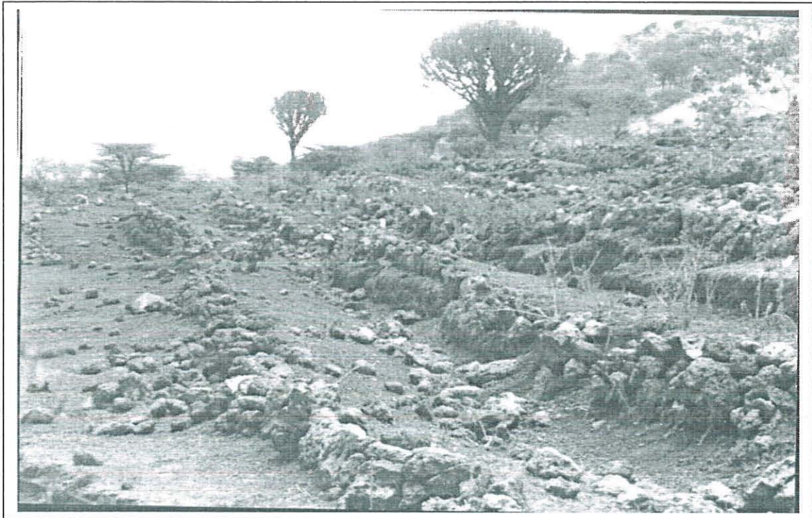
Figure 1. Hillside terraces that lack maintenance work
