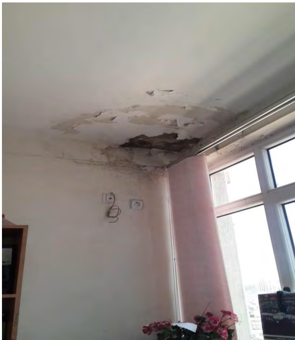
Fig 4.9: – Ceiling leakage
