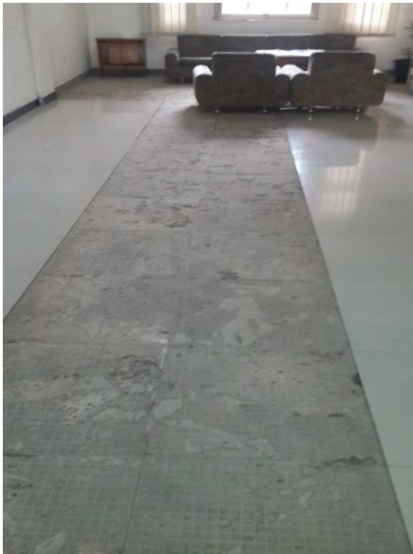
Fig 4.3: – Loosen floor tile
