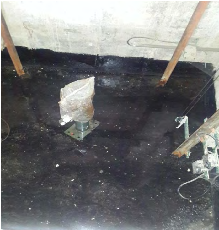
Fig 4.5: - Lift case filled with water
