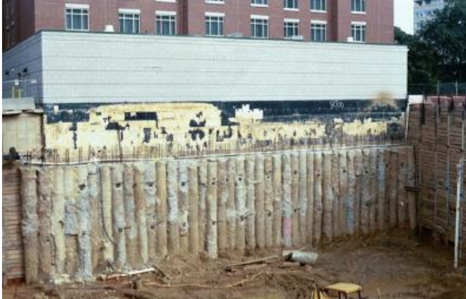
Figure 3 Tangent Bored Pile Wall
