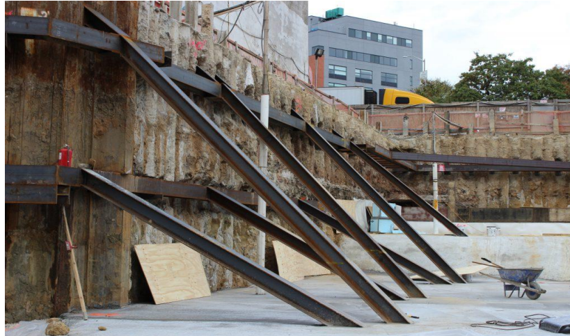
Figure 6 Support for Raker
