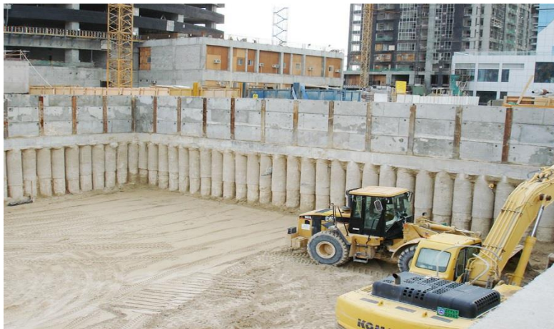
Figure 2 Contiguous Bored Pile Wall
