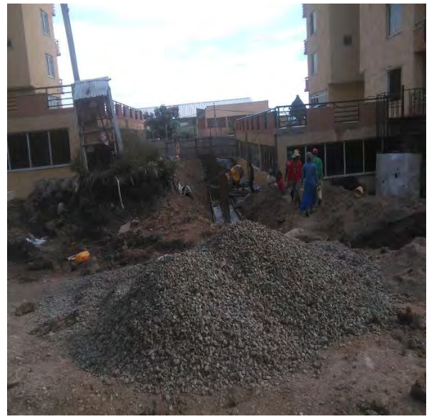
Figure 5.12 Retaining wall construction
