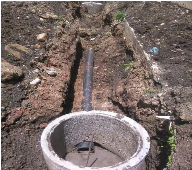
Figure 5.11 Sewer line installation
