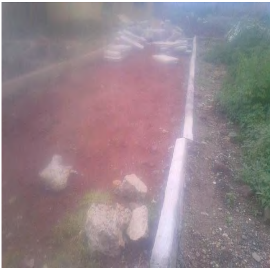
Figure 5. 4 On progress walkway
