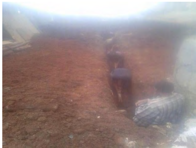
Figure 5.6. Excavation work for sewer line installation
