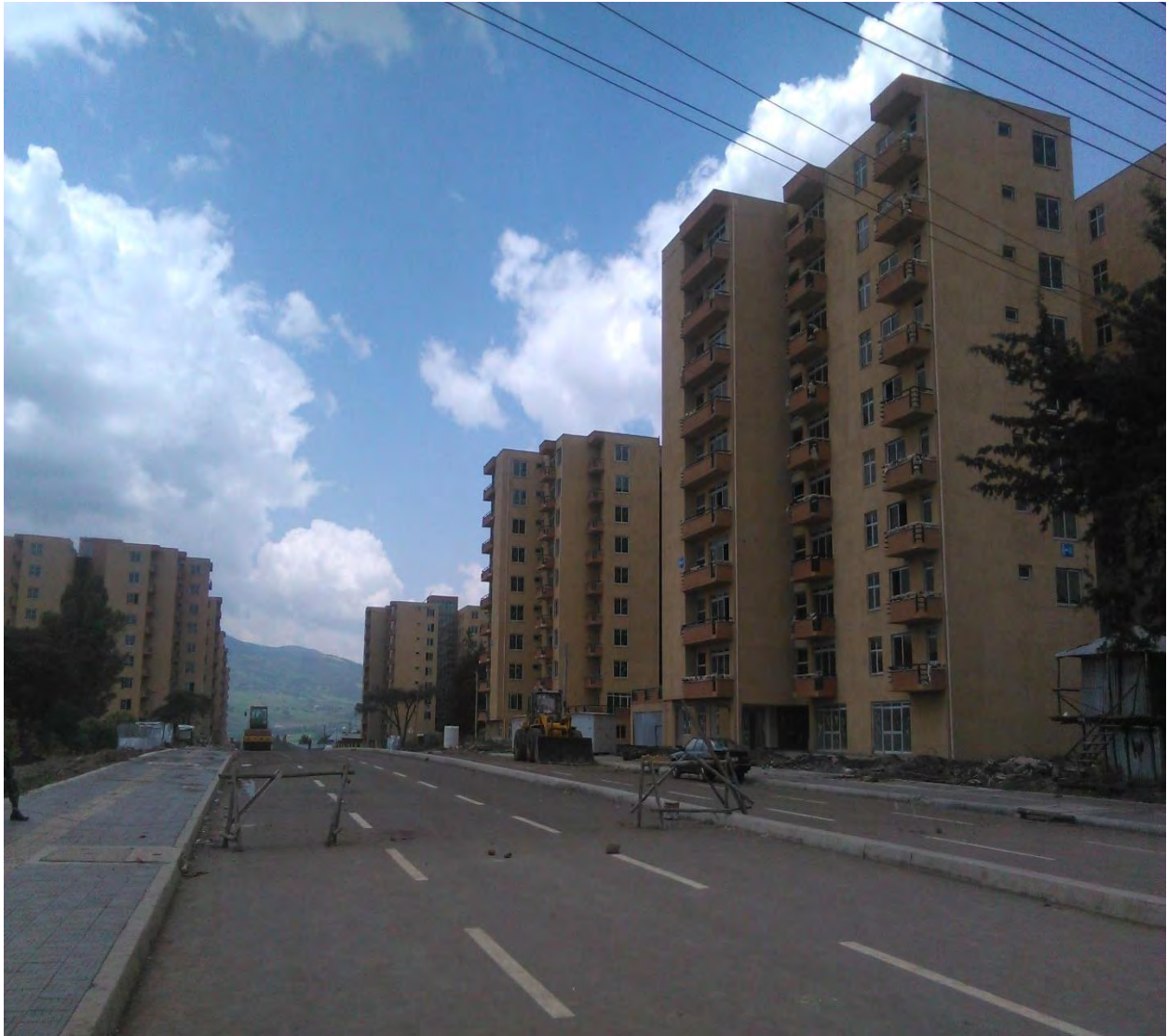
Figure 5.9: Crown 40/60 project site
