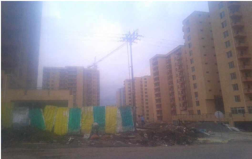
Figure 5.3 Sengatera 40/60 project site
