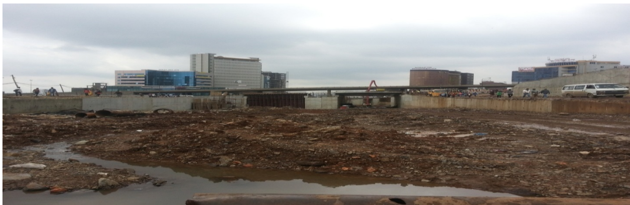
Fig. 4.1 Delayed underpass construction by AACRA at Megenagna
