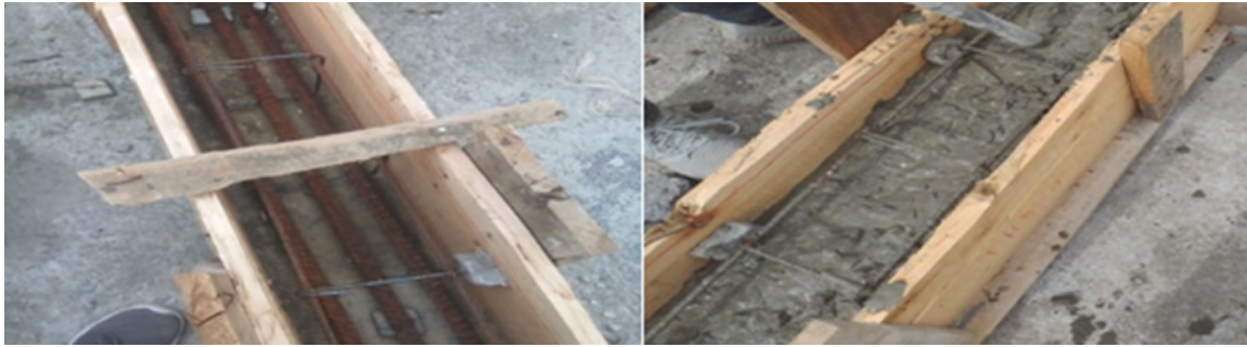
Figure 3-10: Formwork preparation and specimen casting
