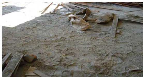
Figure: - 4.10 Wastage of cement due to poor handling, Lack of control & poor storage
