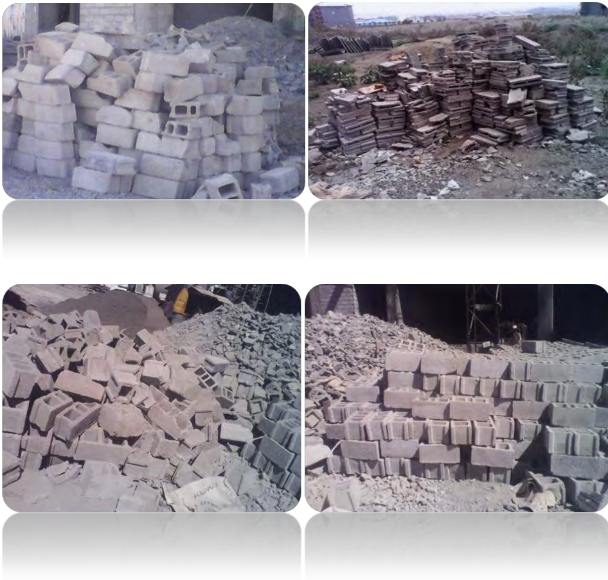
Figure: - 4.1 Wastage of CHB on building construction sites due to poor handling
