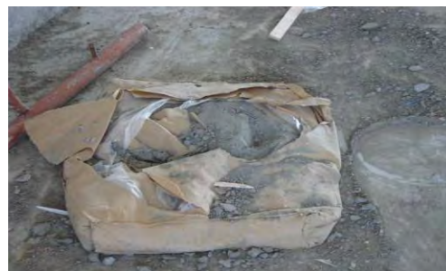
Figure: - 4.10 Wastage of cement due to poor handling, Lack of control & poor storage
