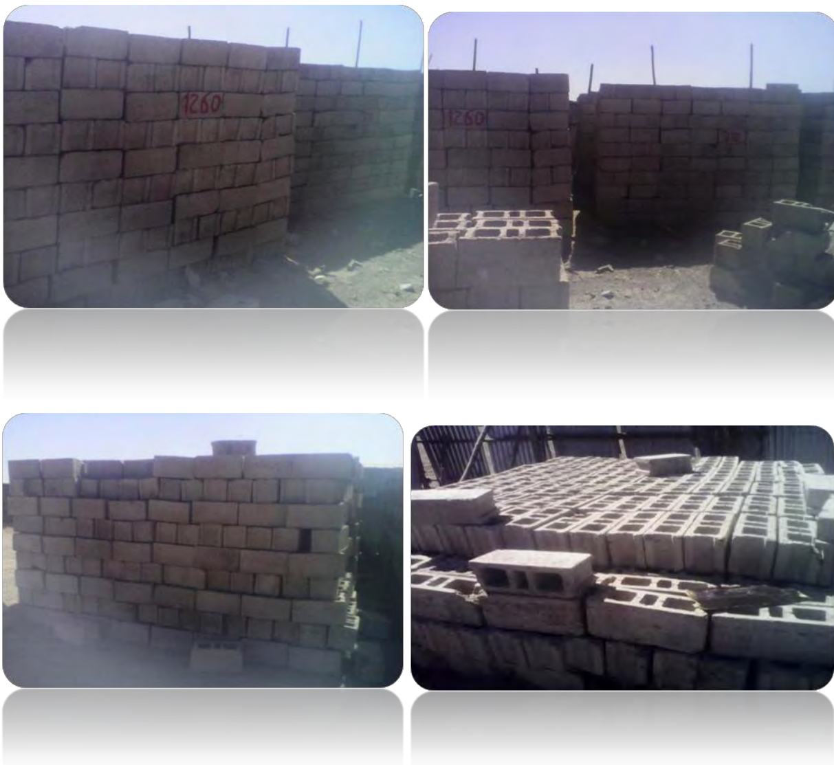
Figure: - 4.3 properly packed HCB on building construction site
