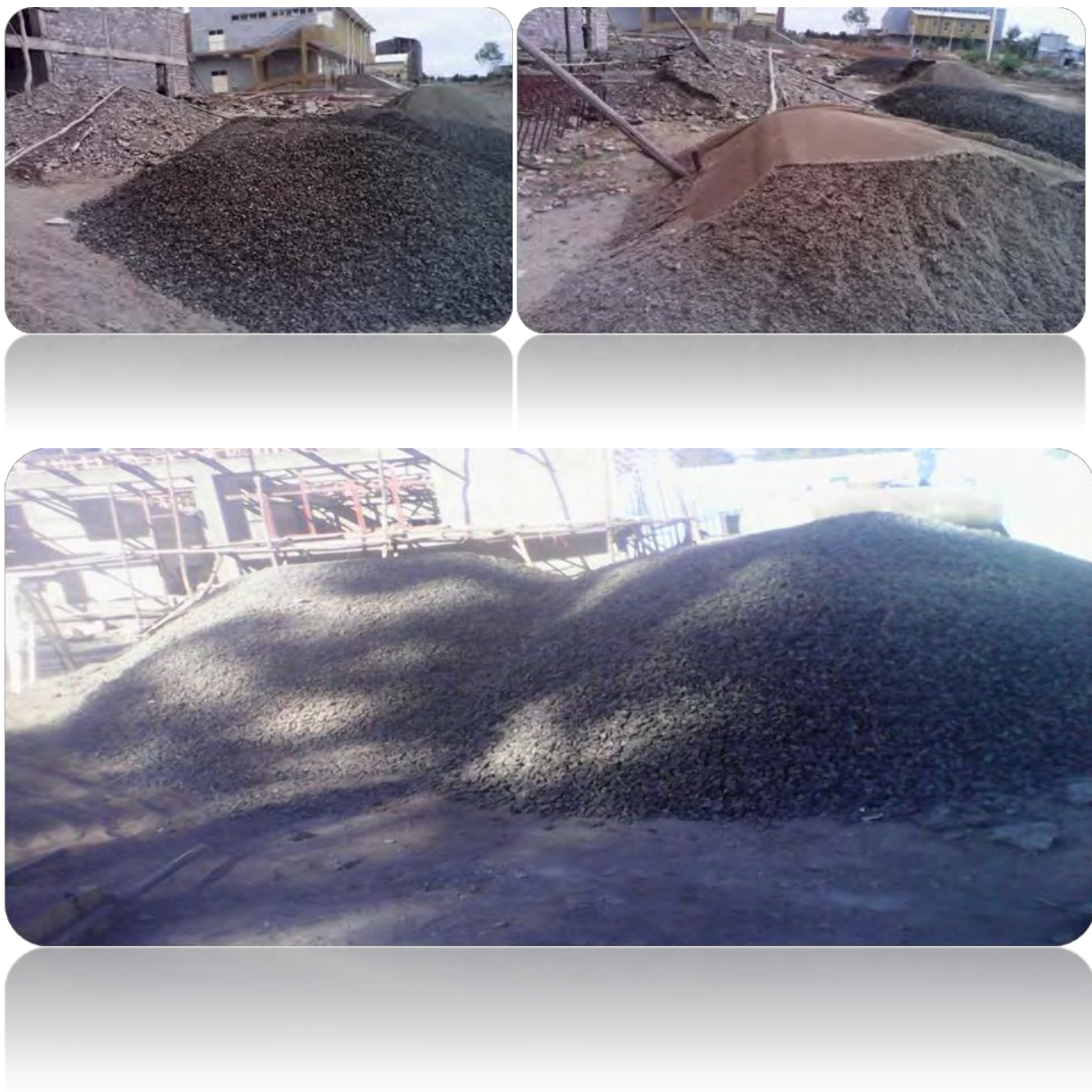
Figure: - 4.8 Good handling of sand and coarse aggregate on building site
