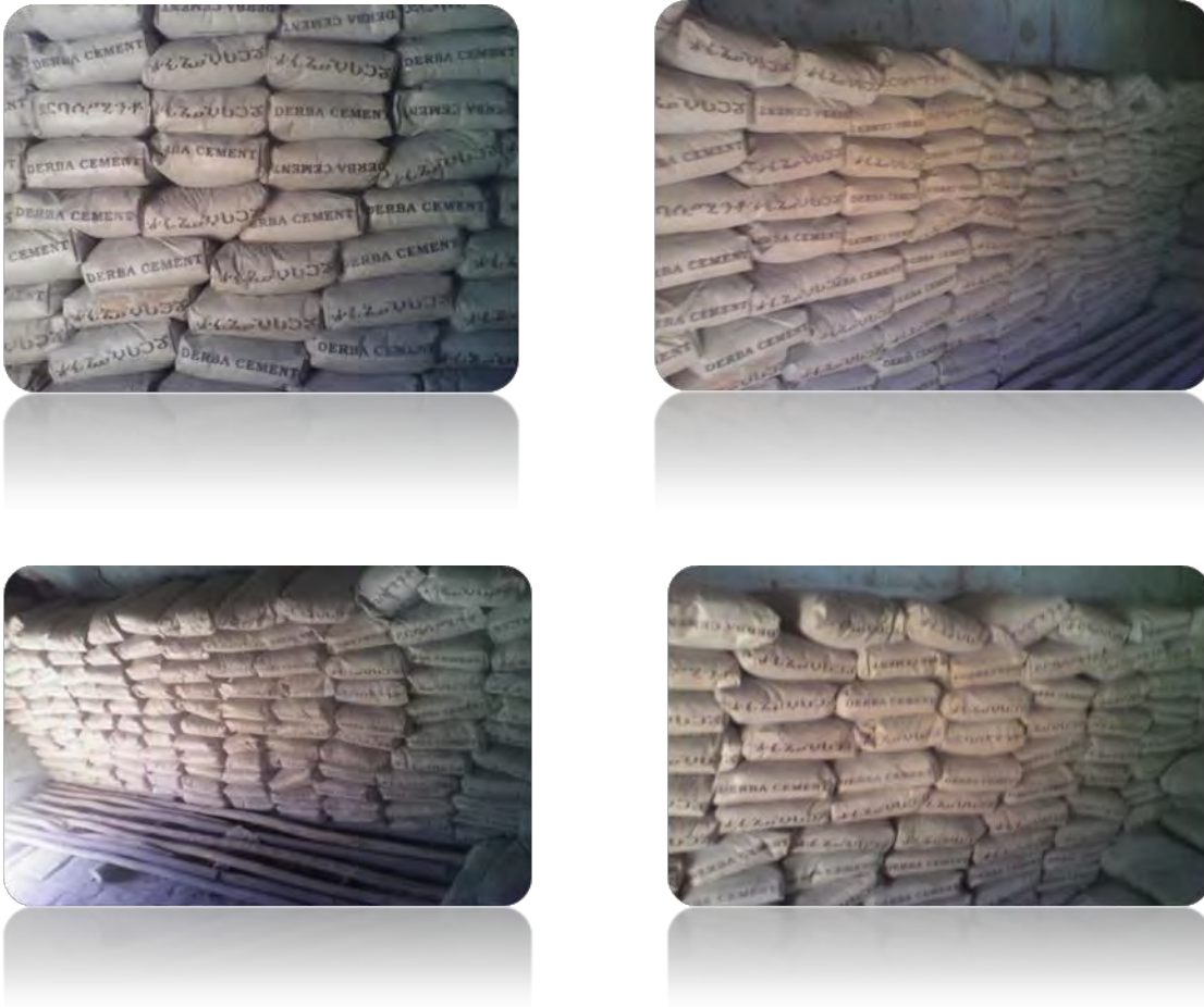
Figure:-4.14 Recommended ways of storing cement on building site
