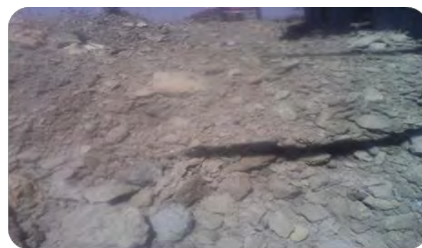
Fig 4.12. Mixing of mortar greater than the required
