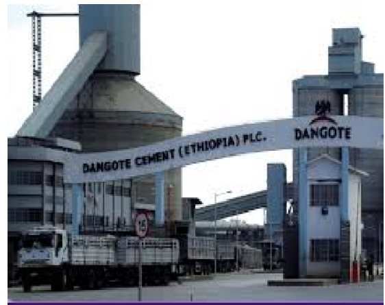
(b) Dangote Cement Factory, Ethiopia, Plc.
