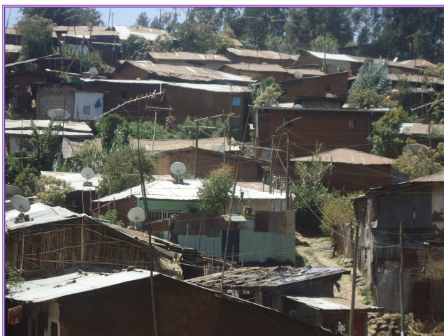
Pic 4.6 houses with limited accessibility.
