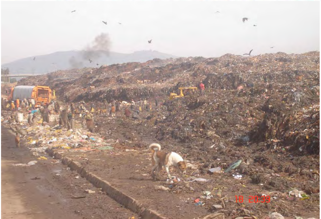
Figure 1.1: Features of Addis Ababa solid waste dumping site 'Reppi'(Photo by sanitation and beautification team of Nifas Silk Lafto sub-city 2007)
