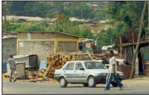
Figure 4.4a One of the toilet and shower facilities built by CARE
