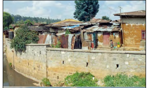
Figure 4.12 flood prevention retaining wall
