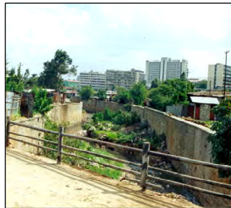
Figure 4.11 flood prevention retaining wall
