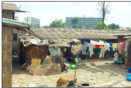
Figure 4.6 Corrugated iron sheet is the dominant roofing material
