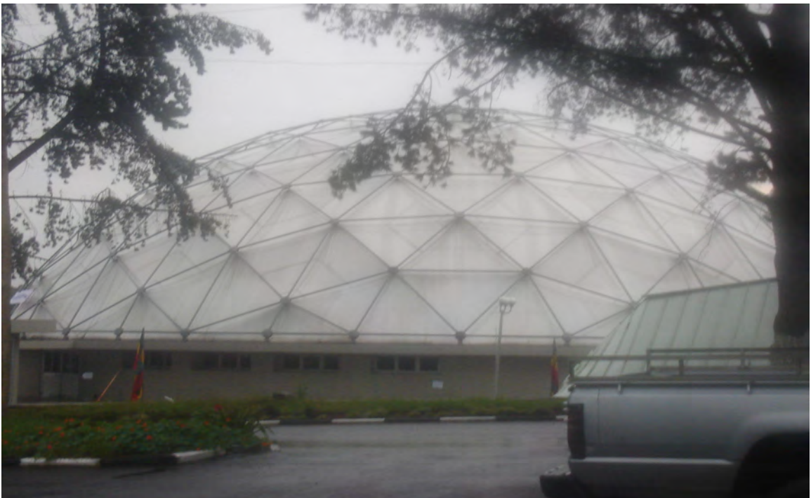
Figure 2.2 Assembly hall in Addis Ababa
