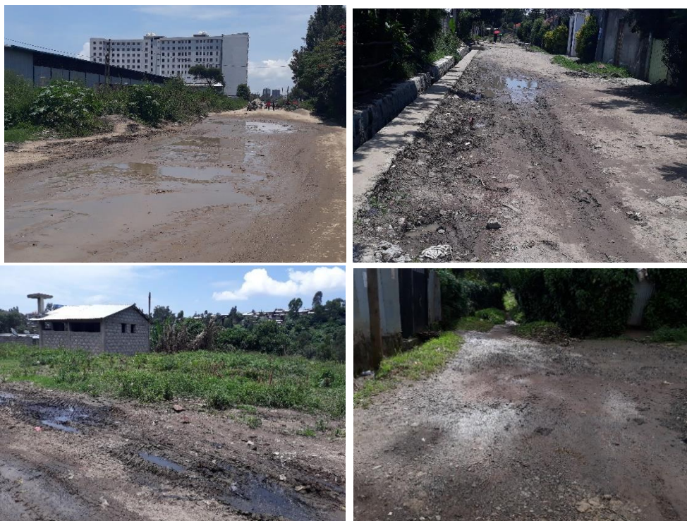
Figure 21: South western part of Addis Ababa with waterlogging problem Jemo(top two ),Lafto(low to the left), and (lower right)Kolfe Keraniyo. (Source: photograph taken by the author on August 2019)
