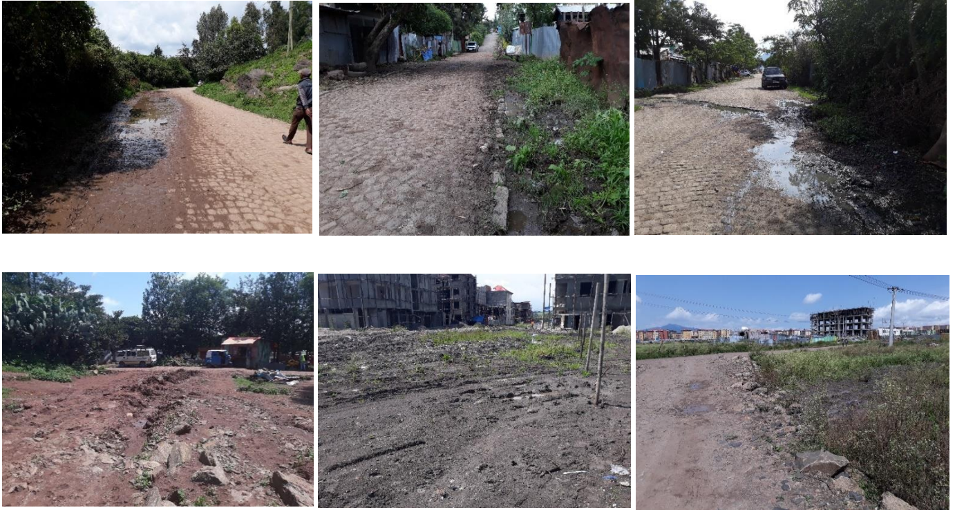
Figure 22: Southern part of Addis Ababa with waterlogging problem Akaki Area(top 2 on the left) kality area(top on the right) and (Bottom 3)Tulu Dimtu area. (Source: photograph taken by the author on August 2019)
