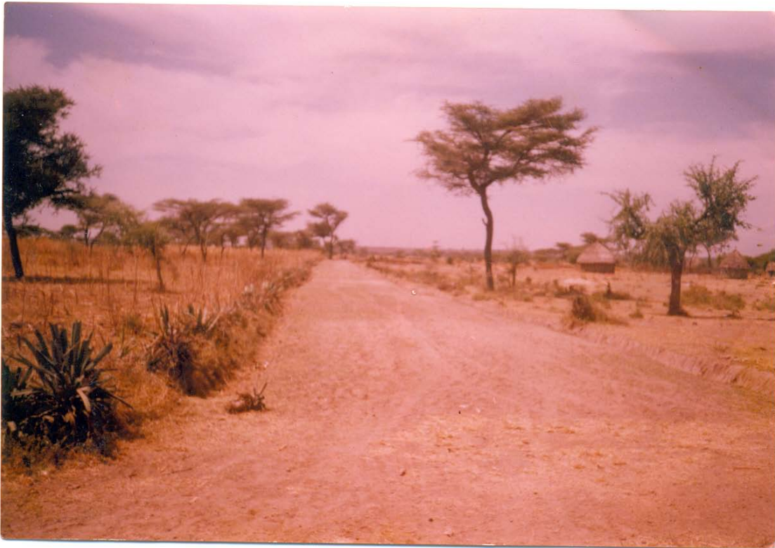
Figure 5: Road constructed or maintained in Chetu Getu in 2006 by PSNP Public work participants
