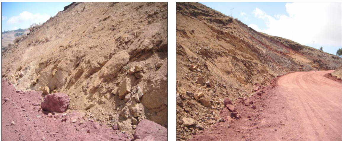
Plate 4.3 small scale landslide along road cuts (1022053N, 548200E UTM)
