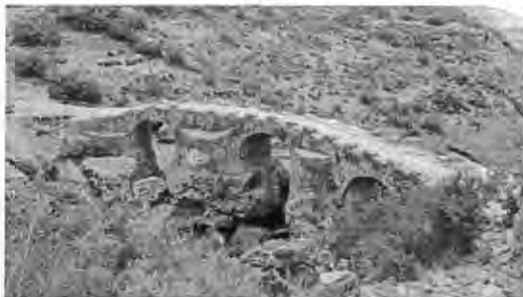
Figure : The Bridge at Debre Libanos (Source: own survey)
