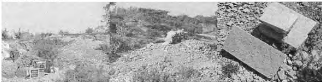
Figure : Mechanical and manual masonry extraction near the bridge at Debre Libanos
