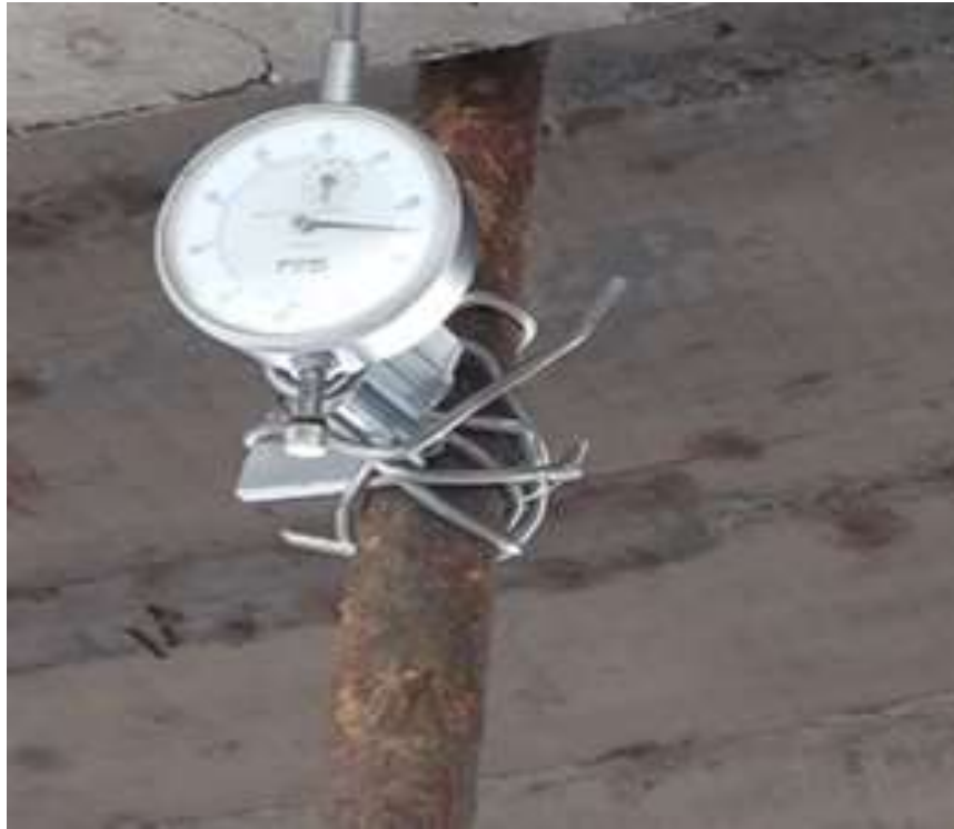
Figure 3.6 Installed deflection measuring tool at mid span of the bridge
