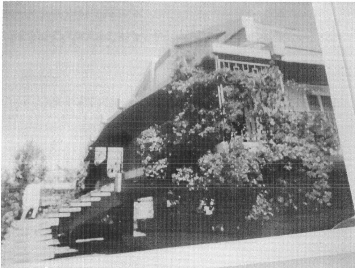
Figure 11: Villa Yilma Déréssa , built by Arturo Mezzedimi in 1960s( After confiscation in July 1975, the Villa is serving as the Embassy of Niger) 1361
