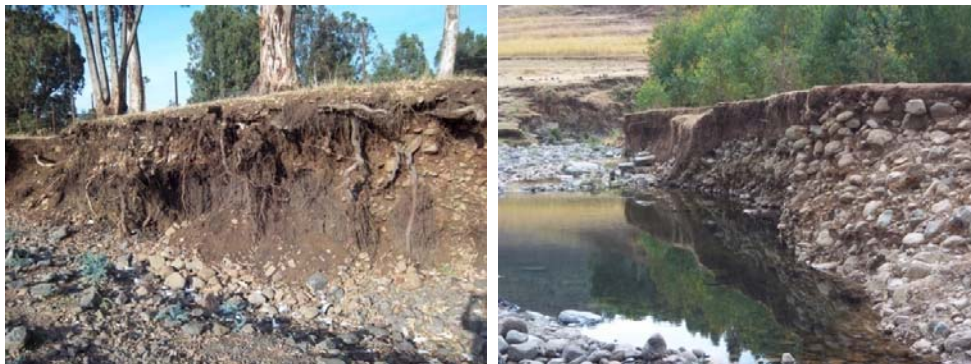
Figure 12. Photo showing existing situation of river banks (taken by the author)
