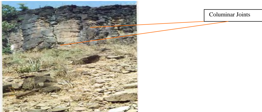
Fig 3.4 Columnar Jointing and Block faulting of the Acidic Lava (photo taken on a Steep Wonji fault escarp at Bilen
