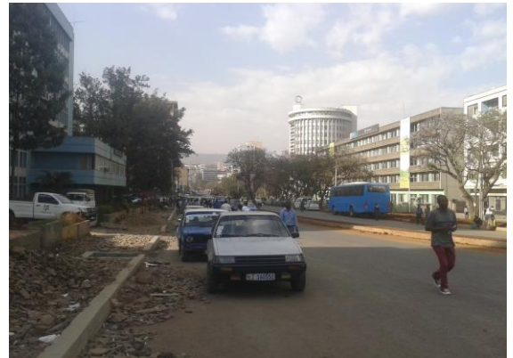
Fig 62: - shows the cracked walkways
