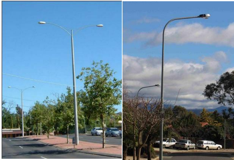
Fig 10:- shows an example of lighting on the street.
