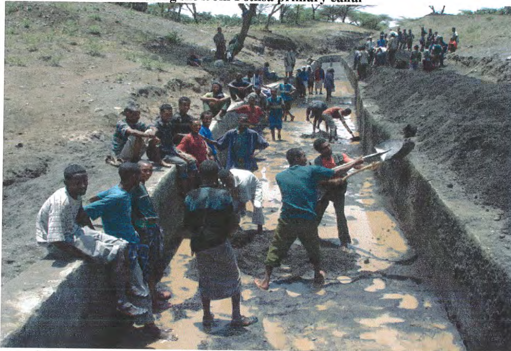
Plate 5.1: Farmers removing silt from Fokisa primary canal
