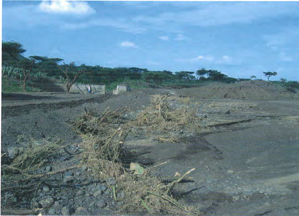
Plate 5.5: Traditional approach canal over modern diversion weir at Fokisa
