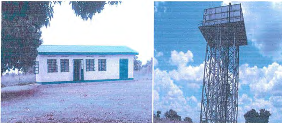
Figure 5.4: Office block constructed by ACCL and 150 cubic meter elevated steel tank at ATC
